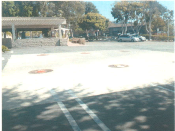
Photo #3: The study site USTs
